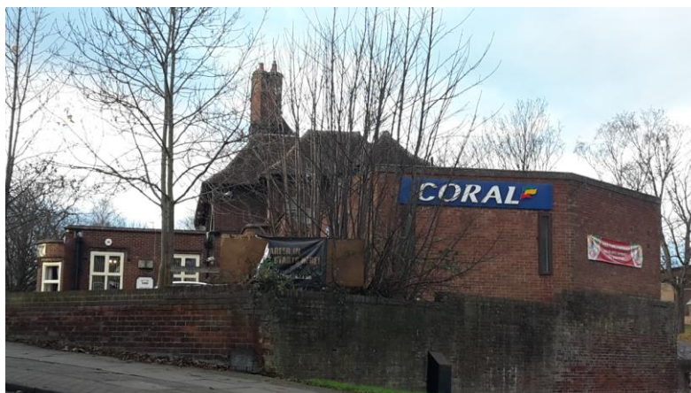
Example of Betting Shop– Durham Road / Darlington Lane
